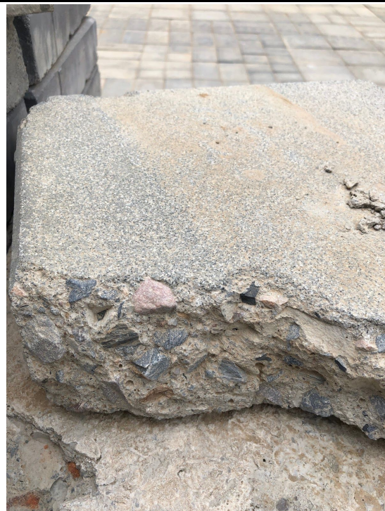
20 mm aggregates used. (against the IS standard). Top layer is non existent
