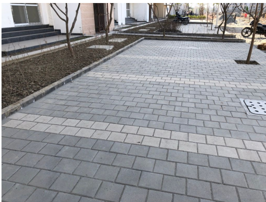
(car parking area)
