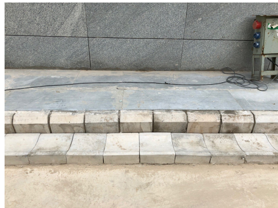
(curbstones must be fixed with jointing mortar)
